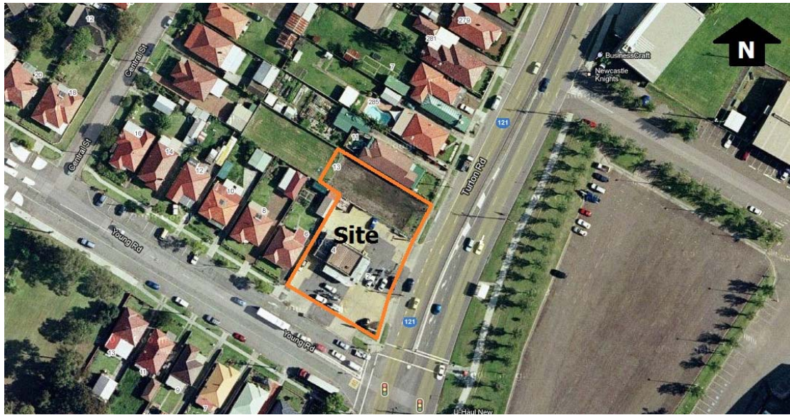
Photograph 1 – Site viewed from Young Road
